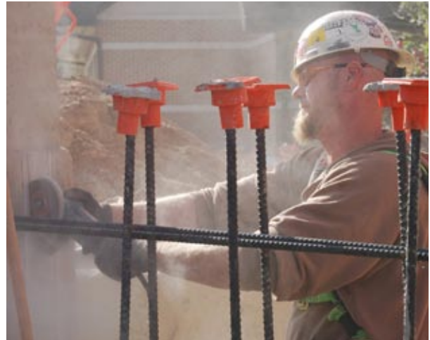
Grinding concrete on one of the pillars.
